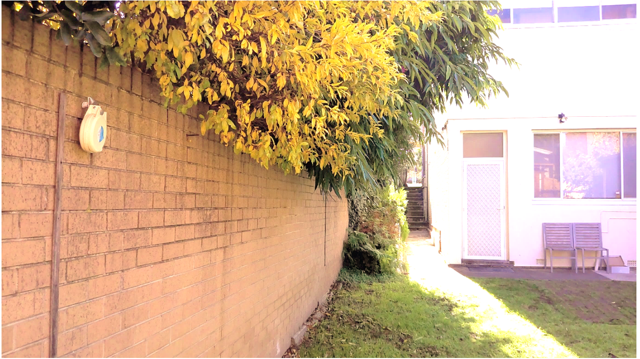
Figure 3.5 – View of subject site from rear looking north
